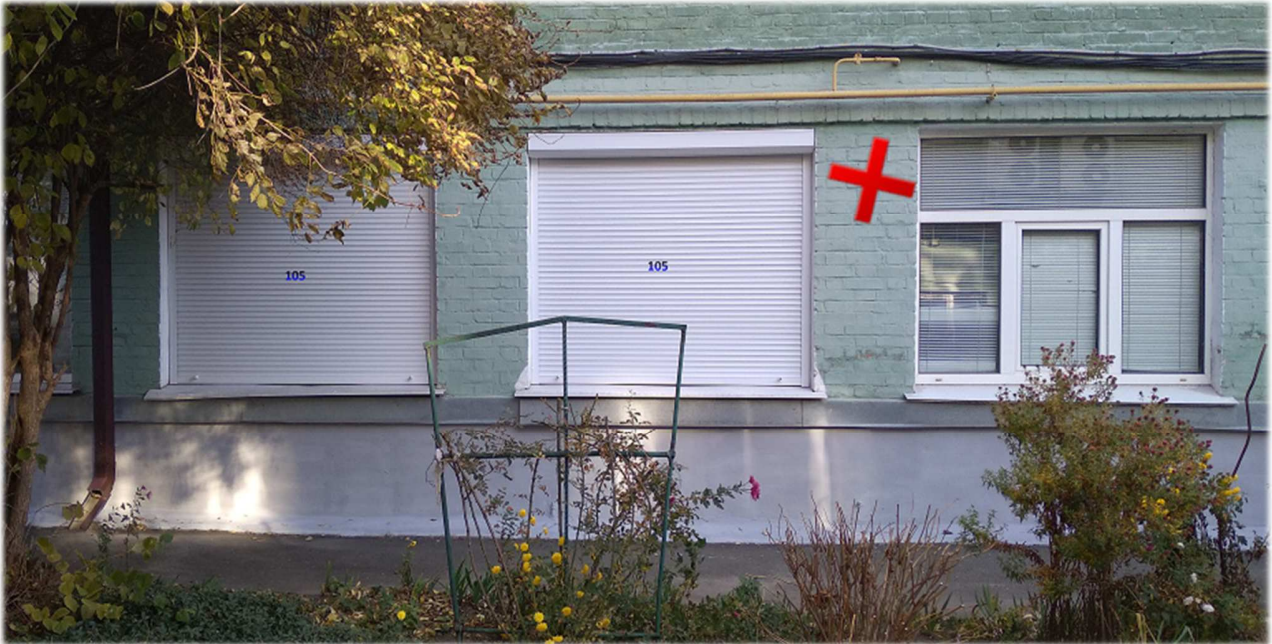
Room 105 (Training Room) – Place of AC external unit installation, street view
