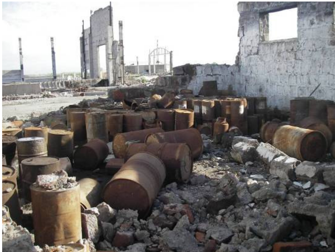
Figure 8.2 Drums with POP's and rubble
