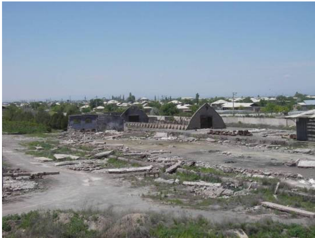
Figure 8.1 Former governmental storage facility and distribution centre for fertilizers and pesticides
